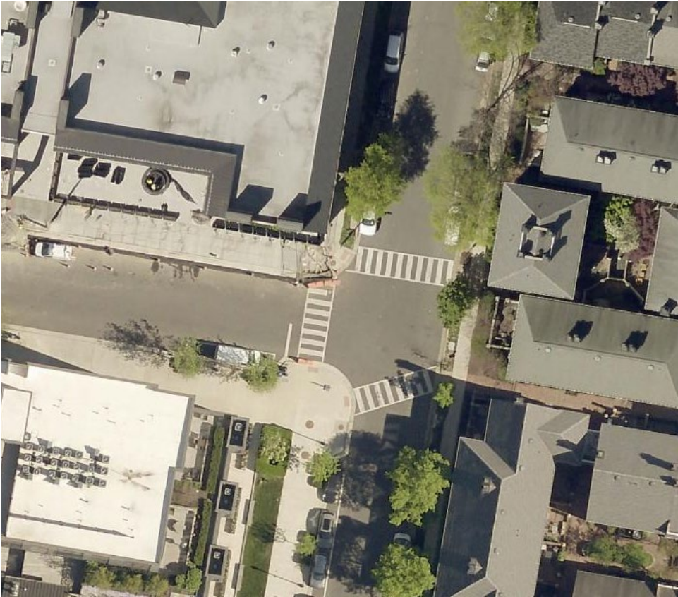
Attachment 1: Location First Street and Pitt Street
