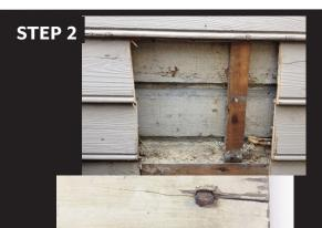
Using clues such as the siding profile and the type of nails used, Staff makes a determination on the age of the siding.
